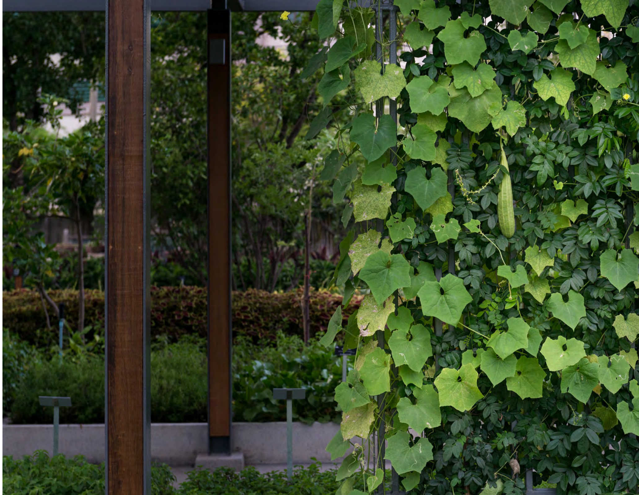
Steel and wood were used to create a 'light' structure that would support the growth of vines in various sunlight conditions.
